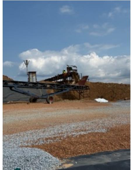
Cell 5. Stacking started and aggregate protective layer on the collection pipes
