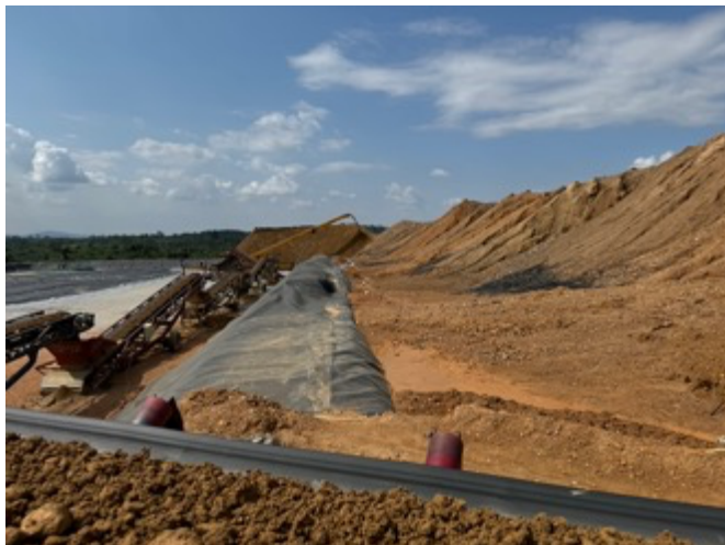
Cell 5. In-filling the gap to Cell 4 for continuous stacking
