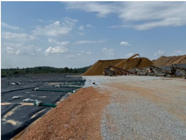
Pad 5 preparation of the leaching process, aggregate layer has to be laid to protect the liner and the collection pipes. Stacking has commenced – getting production moving
