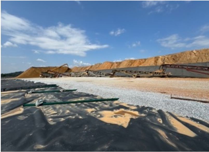
Cell 5. Stacking started and aggregate protective layer on the collection pipes
