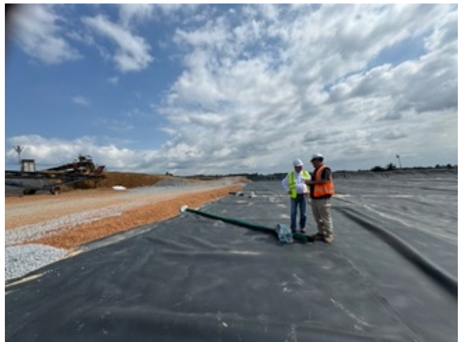
Pad 5 preparation of the leaching process, aggregate layer has to be laid to protect the liner and the collection pipes. Stacking has commenced – getting production moving
