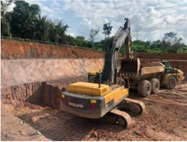
Excess Solution Pond – to be lined
