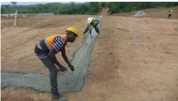
Foundations for Carbon In Solution (CIS) Plant
