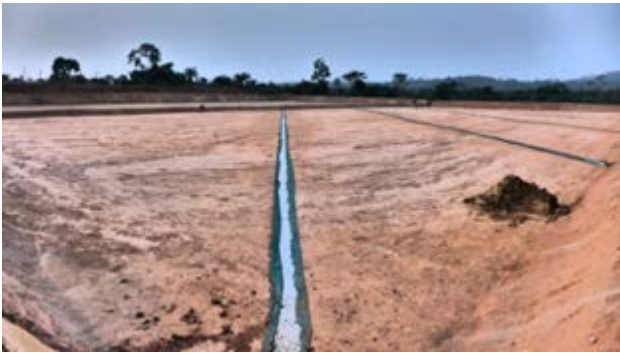
Liner fitted on Cells 1 and 2
