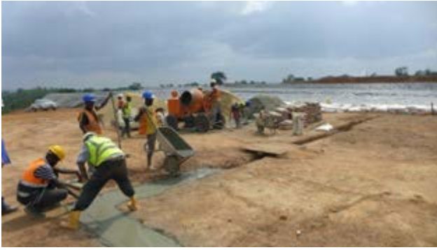
Production of Cushion Layer for Pads
