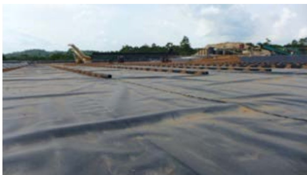
Heap Leach Pad – Cell 1 Collection Pipe
