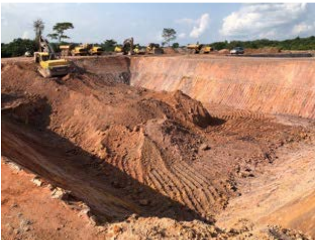
Excess Solution Pond Excavation
