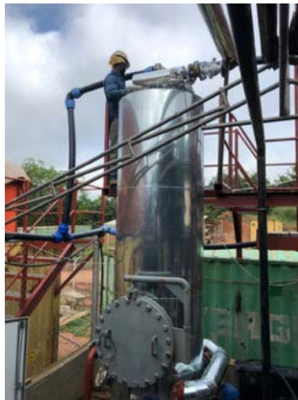
Elution Column being insulated
