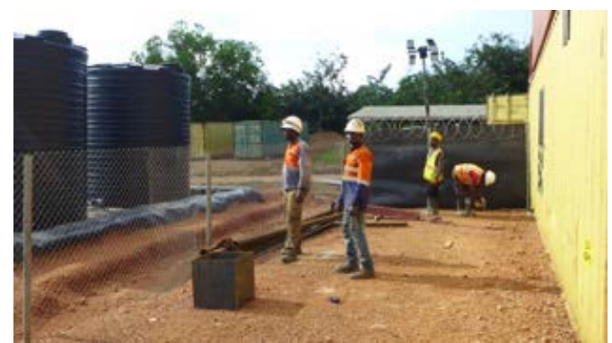
Effluent tanks in bund
