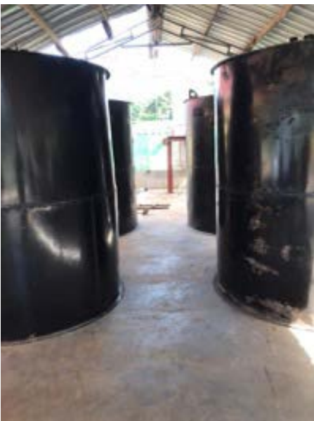
Installation of Elution and Acid Wash Columns and Eluate tanks and Compressor
