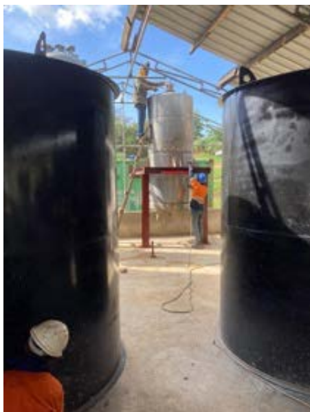
Installation of Elution and Acid Wash Columns and Eluate tanks and Compressor
