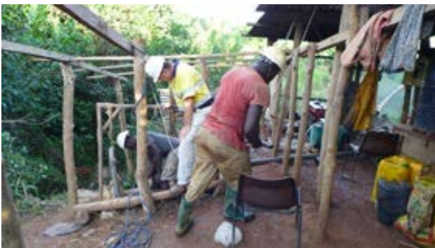
Galamsey Shaft Timber Supports
